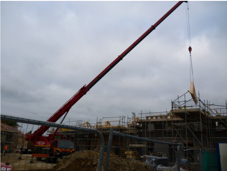
Placing the roof trusses
